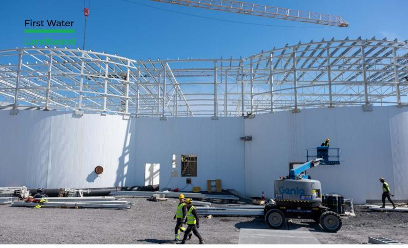
Ongoing work at First Water: use of heavy machinery, piping, and tank assembly are taking place in parallel during the first construction phase. Photo: Therese Soltveit
