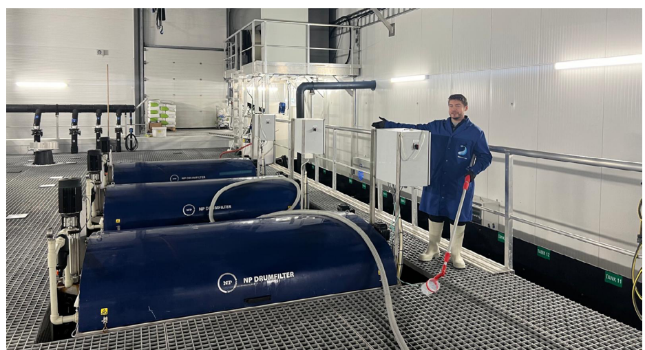
Nanobubbles coagulate particles and increase the performance of mechanical filtration systems. Foto: Moleaer
