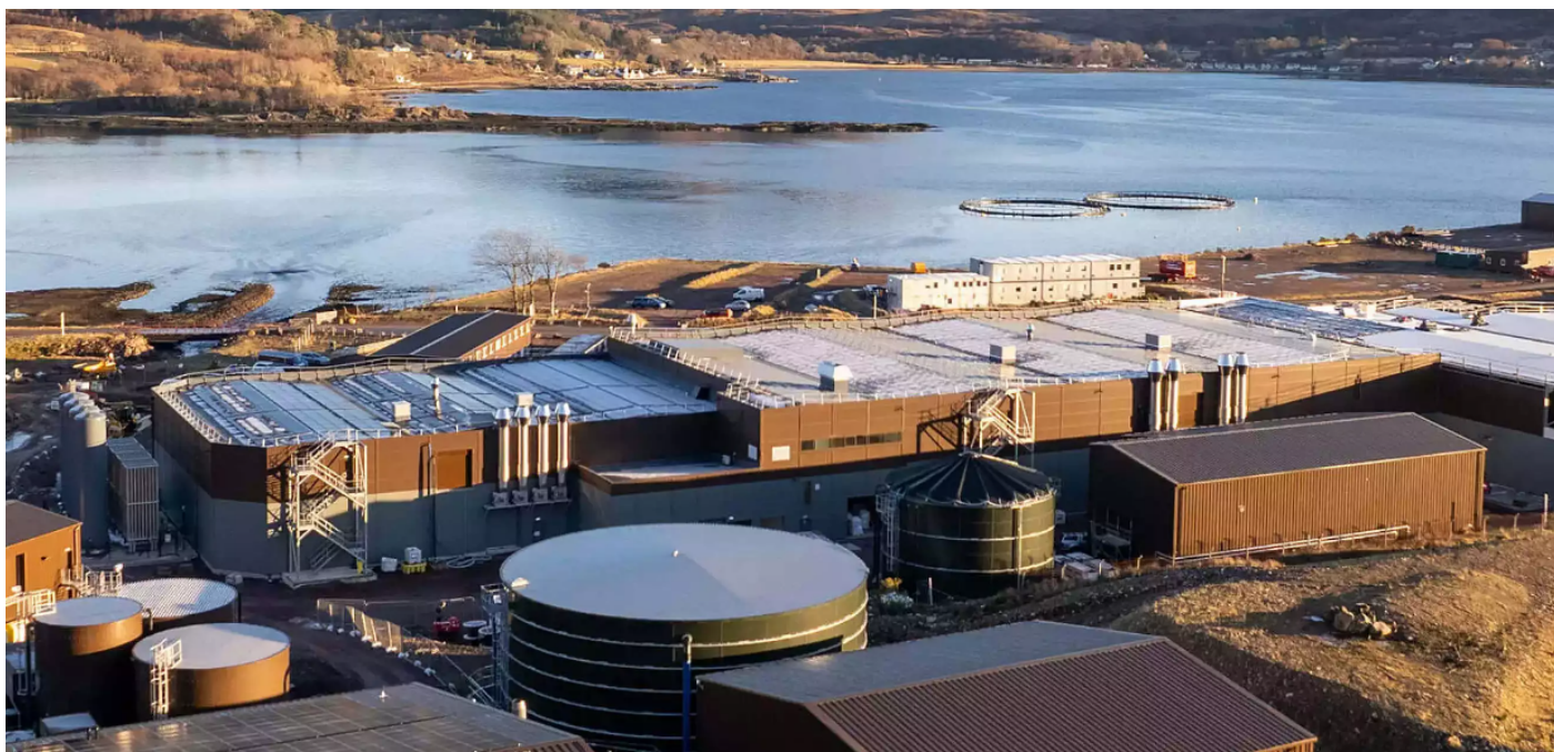
Bakkafrost Scotland's hatchery and post-smolt facility at Applecross, Wester Ross, in the Scottish Highlands. When completed, the RAS facility – which uses technology supplied by Norwegian company Nofitech - will have an annual capacity of 10 million post-smolts with an average weight of 500g.
