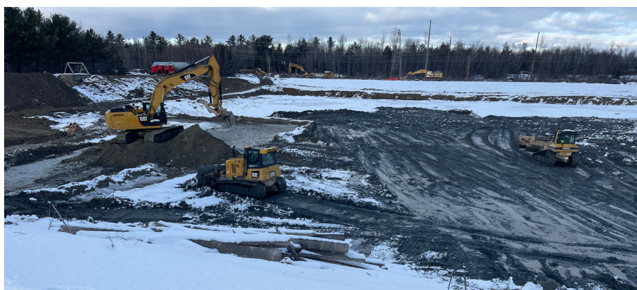
Diggers and bulldozers clear sludge from the floor of a drained lagoon where Great Northern Salmon will build a RAS salmon farm with a capacity of around 7,500 tonnes HOG. Photo: GNS
